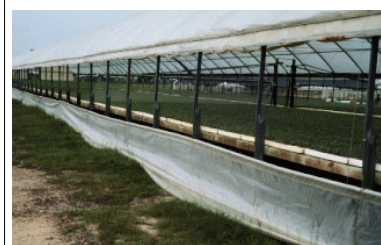
Figure 14. Side vents are needed to achieve good natural ventilation.
