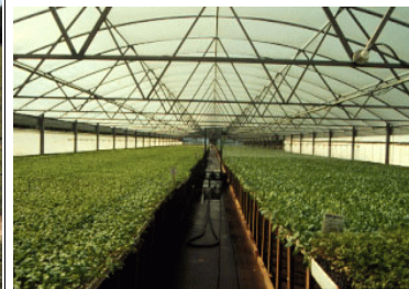
Figure 11. Galvanized steel tubing is often used in constructing greenhouses to be used for transplant production. Steel tubing facilitates maximum light transmittance.
